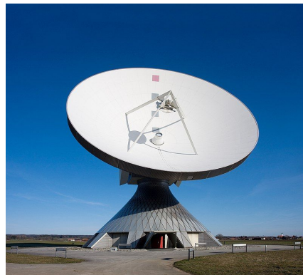
Parabolantenn (Parabolic reflector) 1
